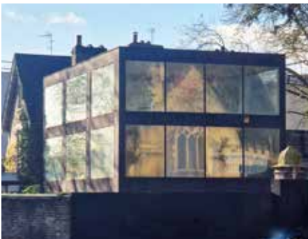
Above 81 Swain's Lane, designed by John Winter for himself, 1967. Now listed Grade II*, it is soon to be sensitively restored and extended
